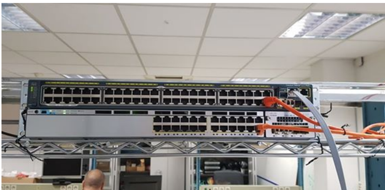
Figure 18 : Installation Switch 3750
